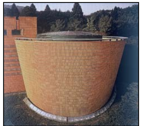
This round building, which uses unglazed terra cotta units, was designed by Mario Botta for the Leeum, Samsang Museum of Art. (Seoul, Korea)
