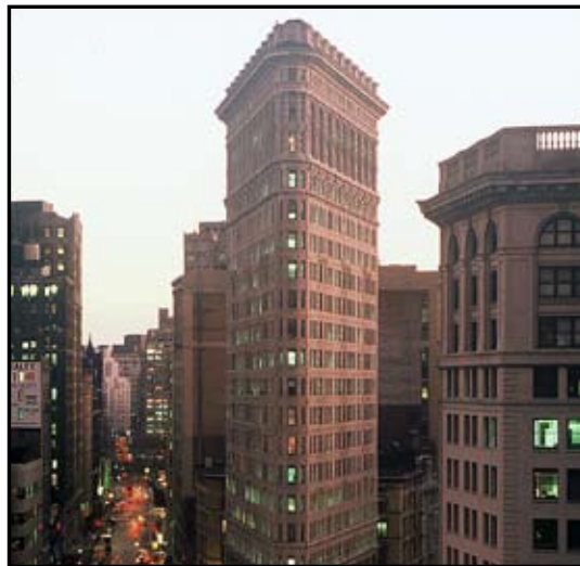
The facade of Daniel Burnham's Flatiron Building from 1903, combines brick and terra-cotta ornamentation. (175 Fifth Avenue, NYC)
